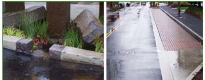
Left: Curb cuts capture stormwater runoff into landscaping where soil layers clean water naturally.
